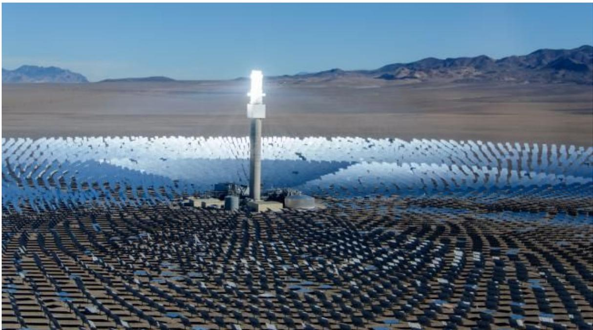
on to the tip of a 195m concrete tower containing tens of thousands of tonnes of a sodium and potassium nitrates mix which acts as a giant battery.
